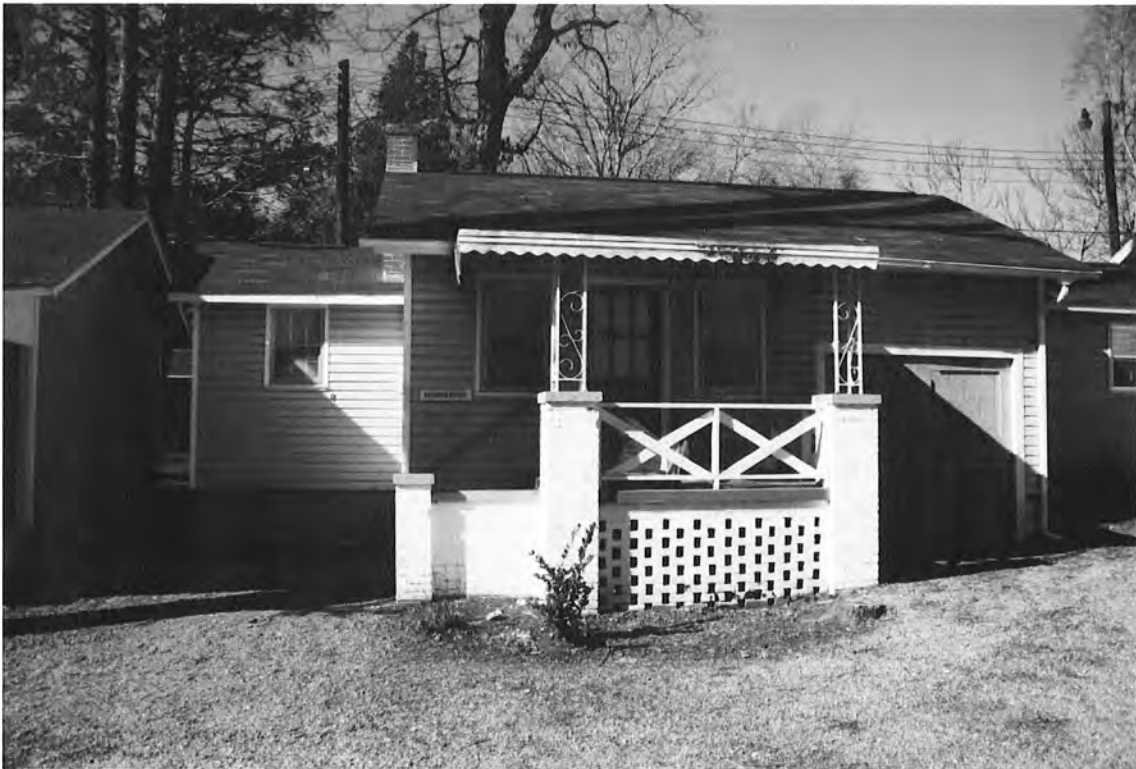
Rhododendron Cottage, 35 Bent Oak Drive, view to north
