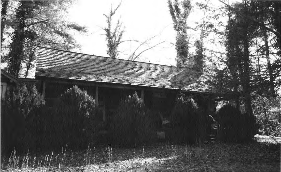
Hiram King Jones House, façade, view to south
