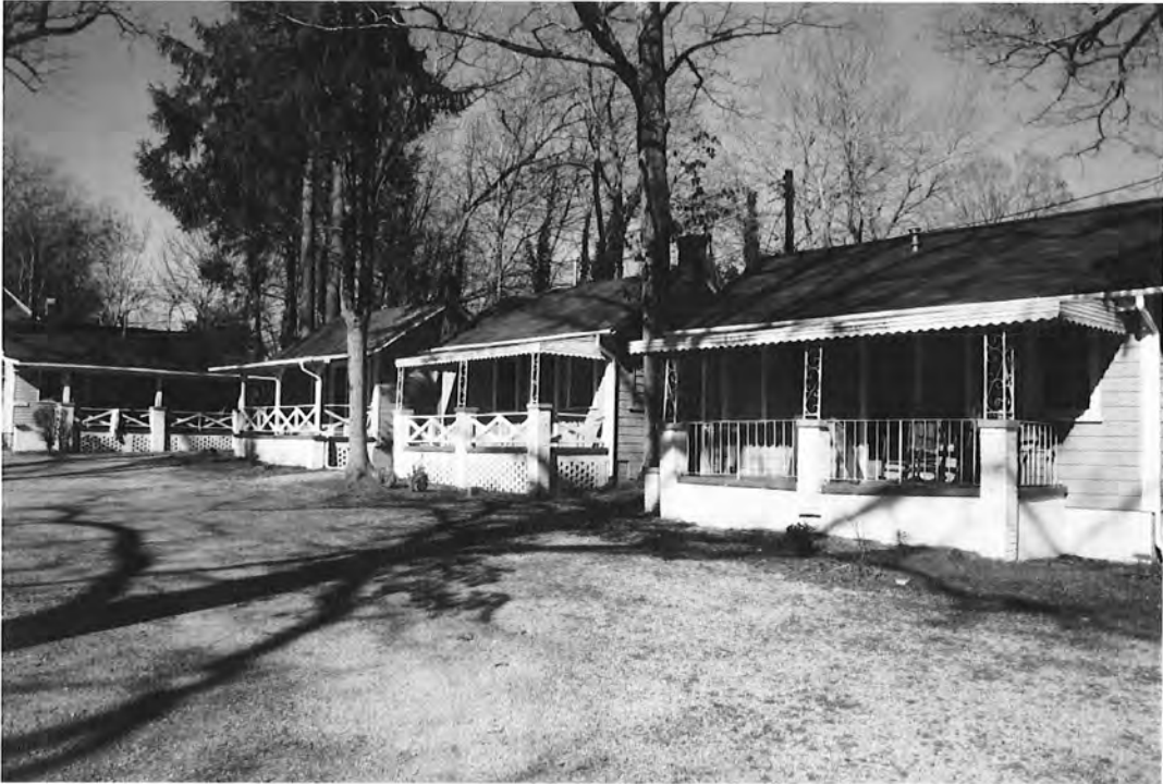
Cottages, 41, 45, 49 and 53 Bent Oak Drive, view to north
