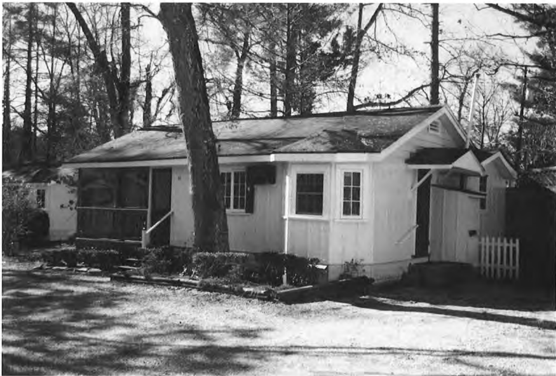
Cottage #10, 50 Ivy Brook Lane, oblique front view to southwest
