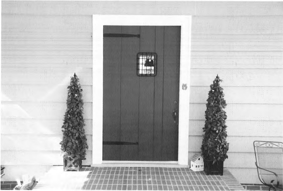
Collins House, front entrance door, view to west
