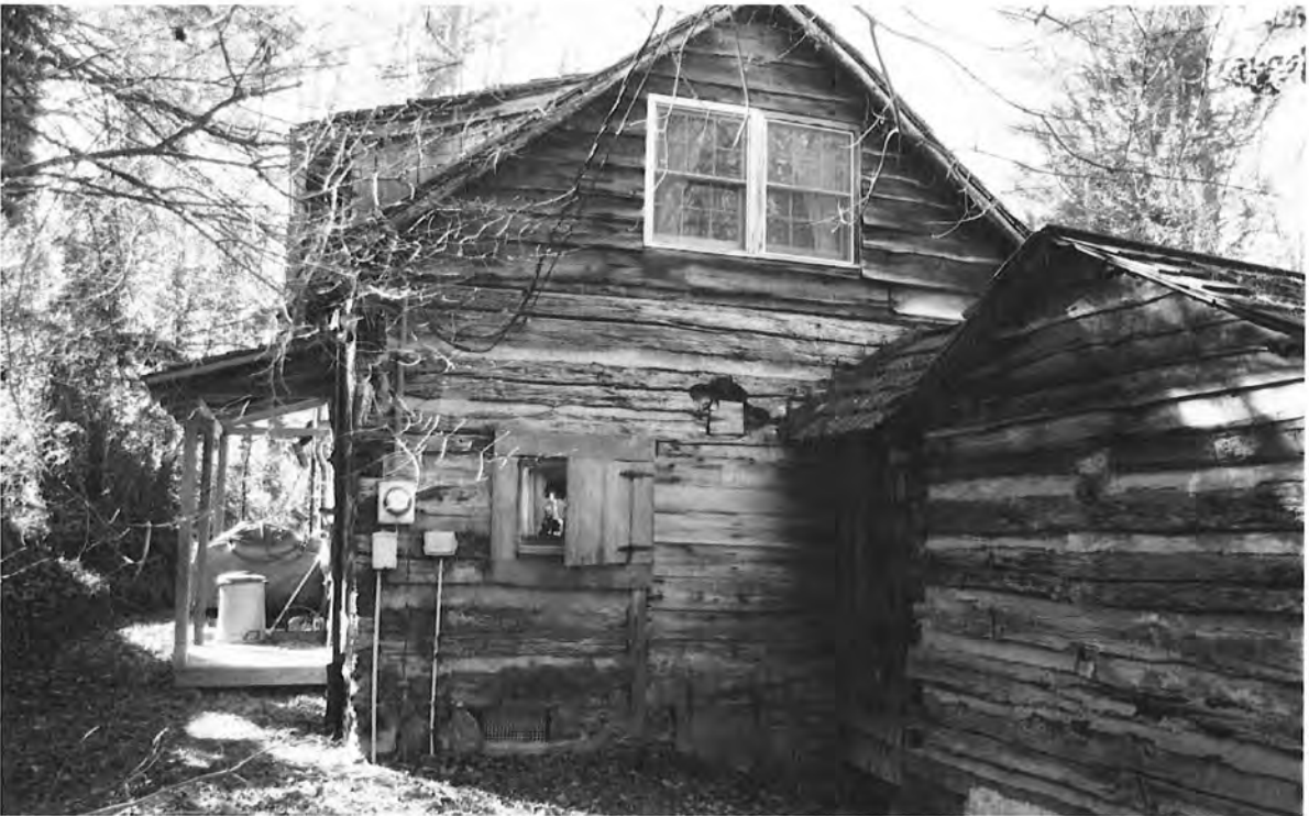
Hiram King Jones House, northeast elevation, view to west
