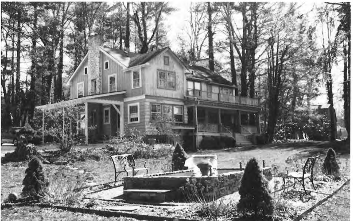
Collins House, oblique rear view to southeast; fountain in foreground
