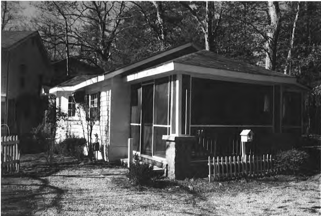
Cottage #12, 22 Ivy Brook Lane, oblique front view to west
