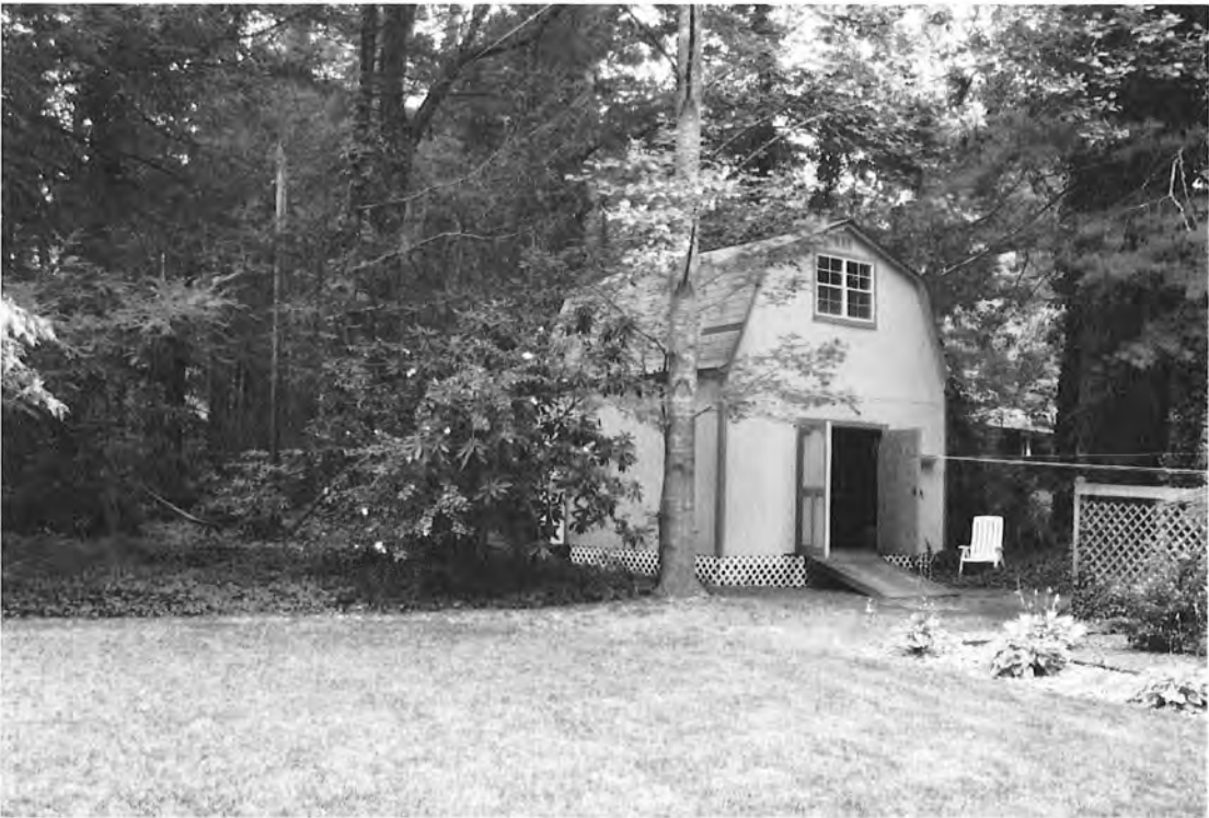
Storage building, oblique front view to southeast
