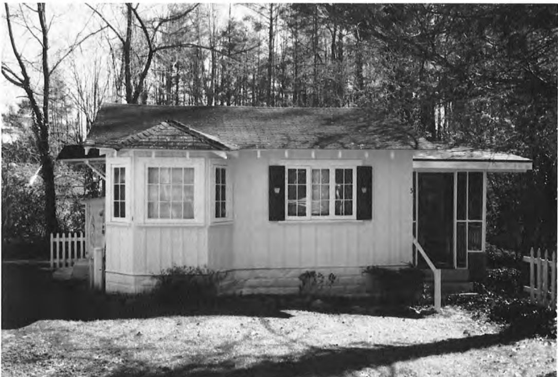
Cottage #5, 96 Ivy Brook Lane, façade, view to southeast
