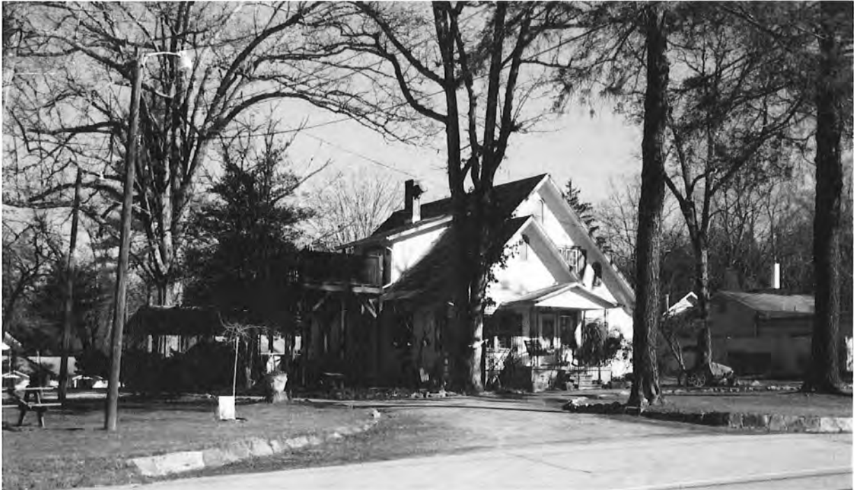
Villa Capri Cottages (former Carolina Court), 920 Greenville Hwy, main residence, view to east
