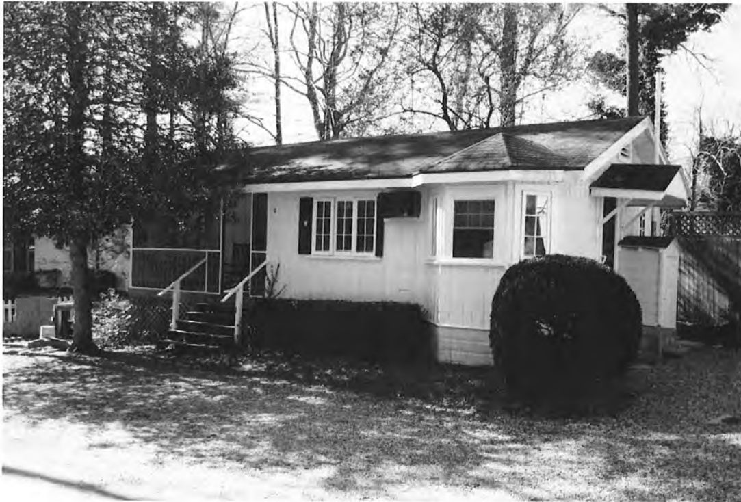
Cottage #9, 70 Ivy Brook Lane, oblique front view to southwest
