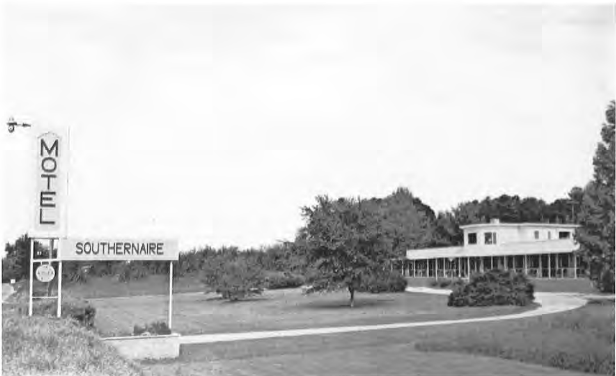
Southernaire Motel (HN 1268), 2990 Chimney Rock Road, postcard view
