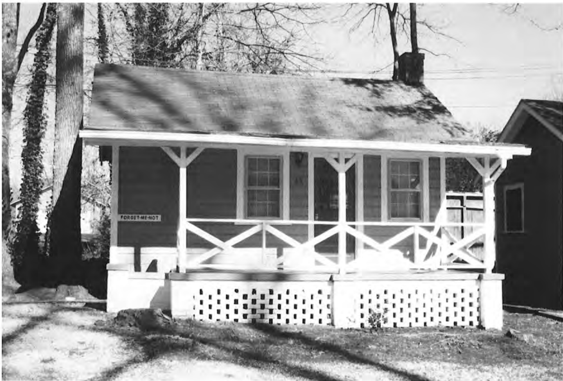
Forget-Me-Not Cottage, 45 Bent Oak Drive, view to northeast
