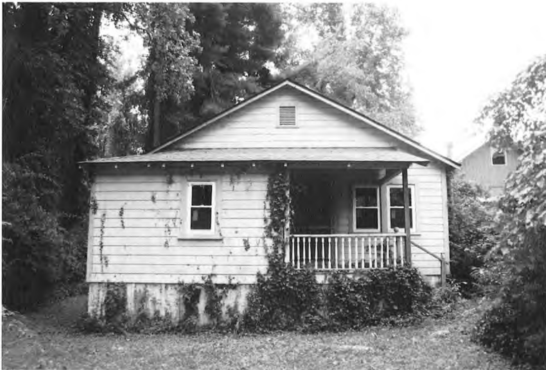
Guest House, façade, view to south
