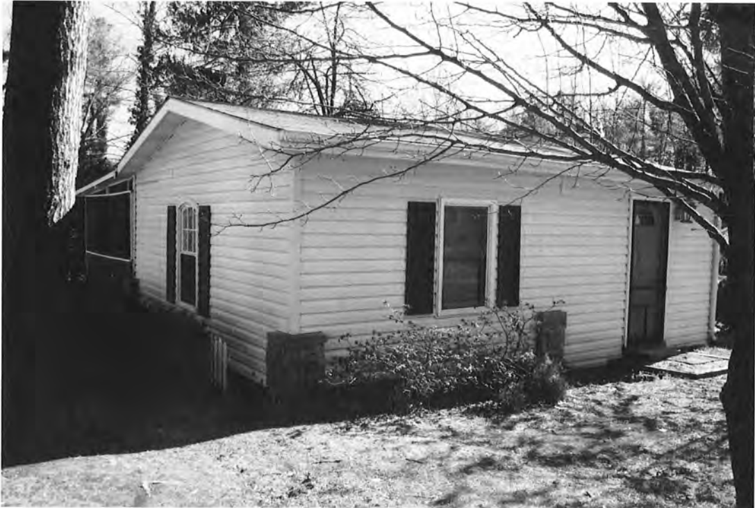
Cottage #14, 139 Ivy Brook Lane, oblique front view to southeast
