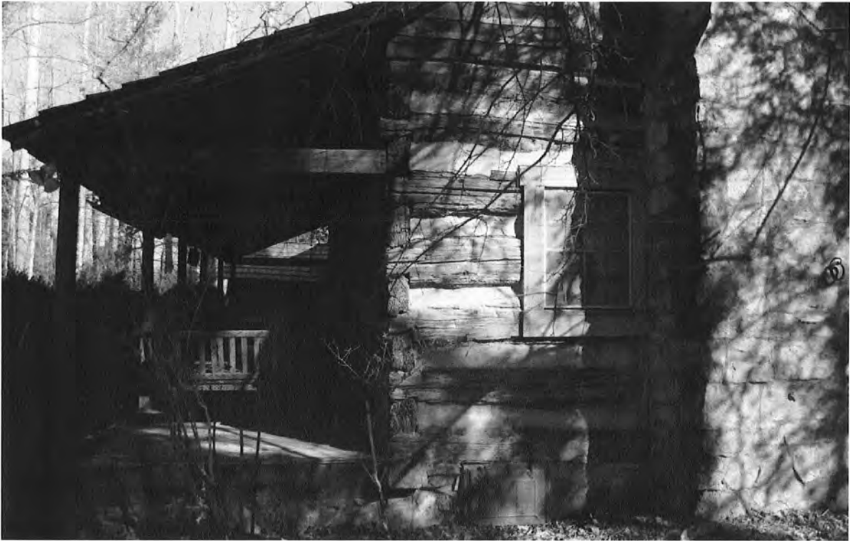
Hiram King Jones House, southwest elevation, view to northeast
