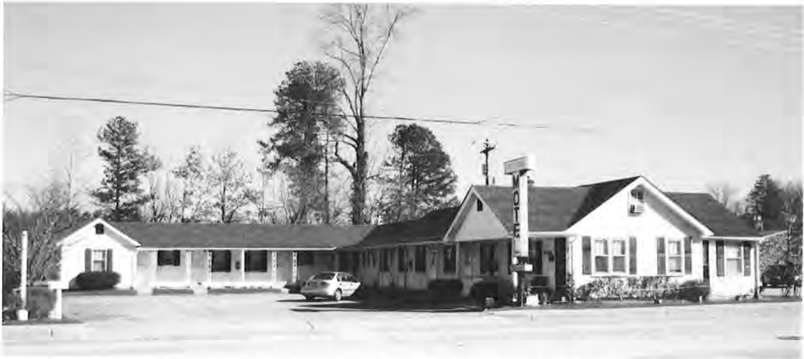
Southwind Motel, 1640 Asheville Highway, view to east
