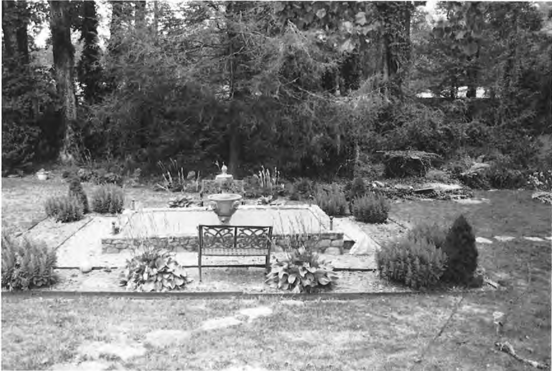
Collins House, foundation, view to west
