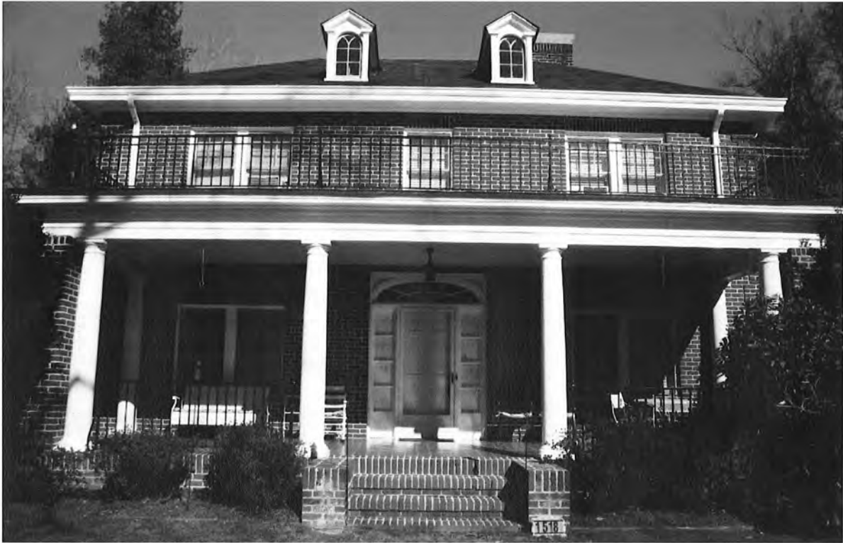
Glenn-Sherman House, façade, view to northeast
