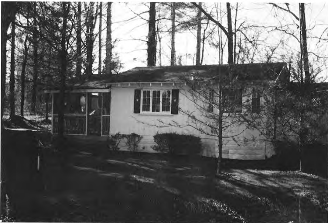
Cottage #8, 46 Drifting Cloud Lane, oblique front view to west
