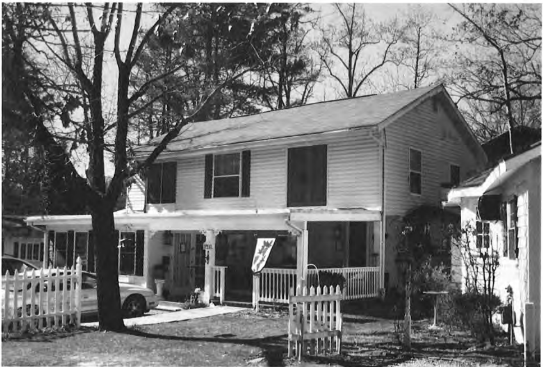
House/Office, 38 Ivy Brook Lane, oblique front view to southwest
