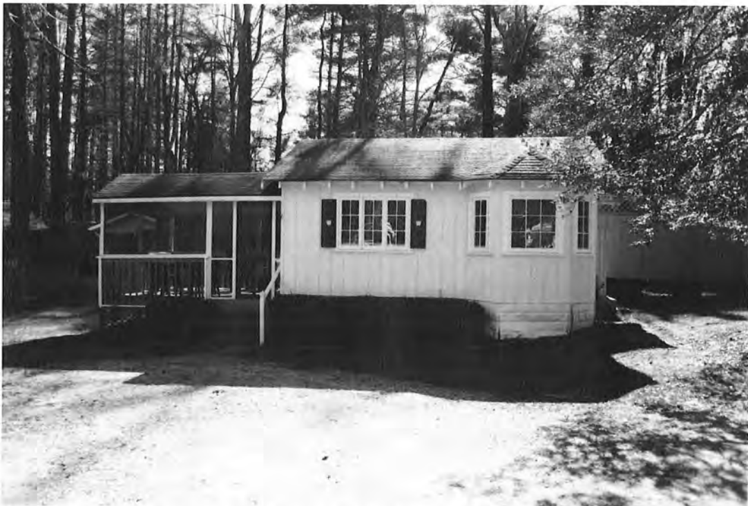
Cottage #6, 15 Drifting Cloud Lane, façade, view to south
