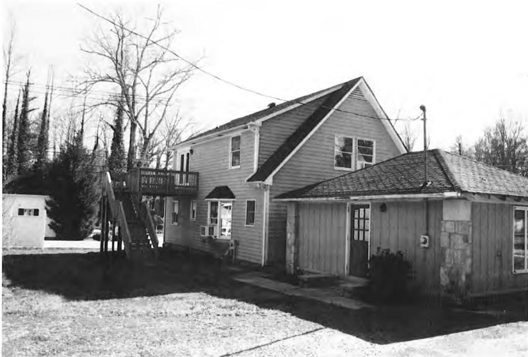
Ivy Cottage (l) and Pavilion (r), 73-75 Bent Oak Drive, oblique rear view to south
