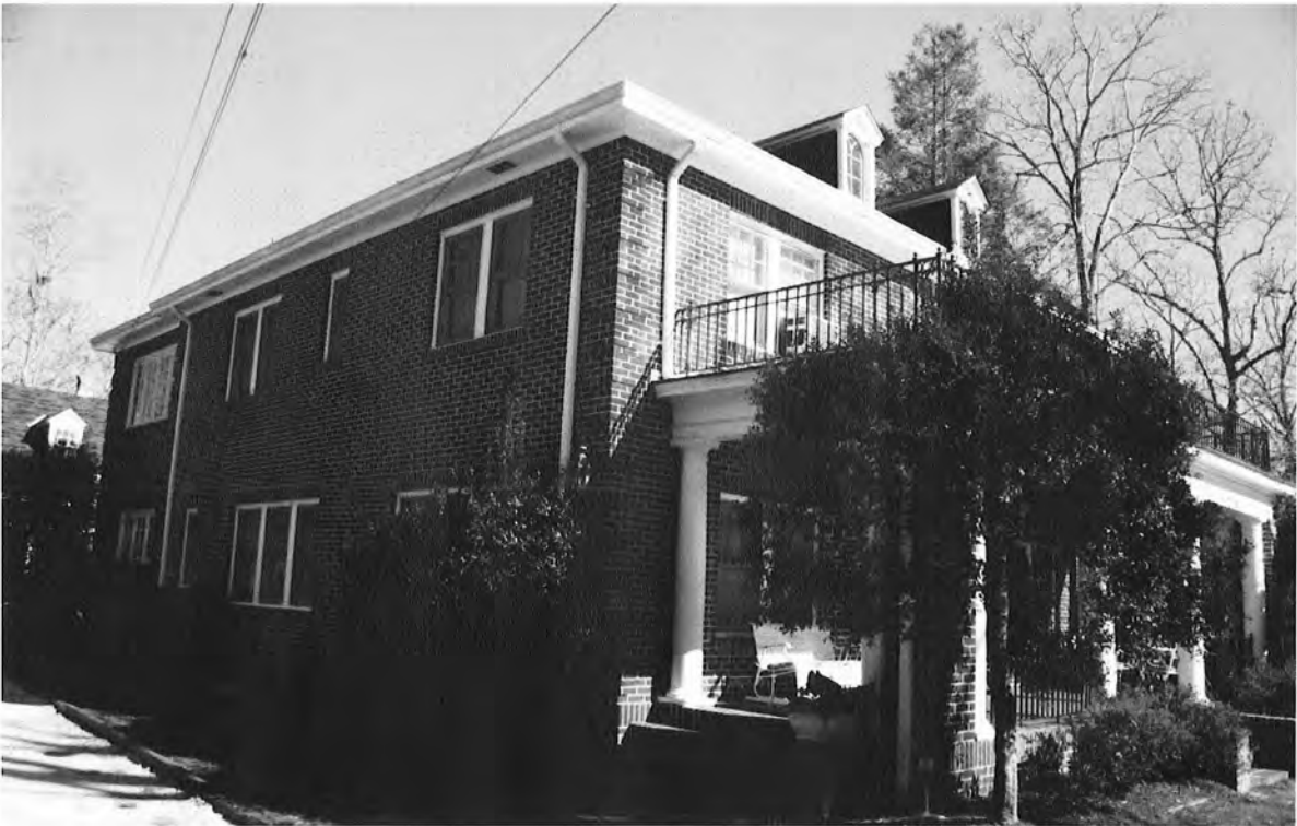
Glenn-Sherman House, northwest elevation, view to east
