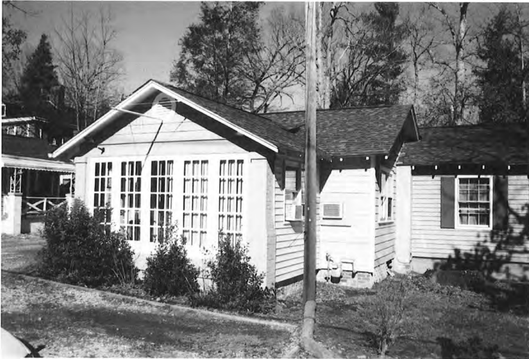
Office, 18 Bent Oak Drive, view to north
