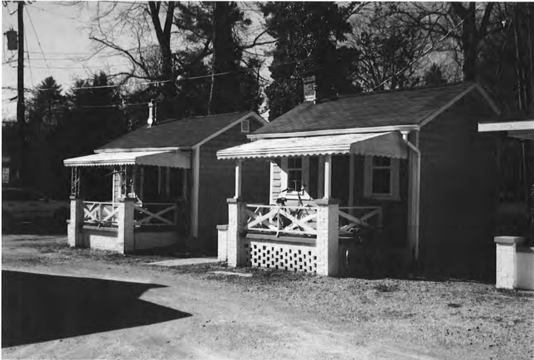
Cottages, 15 and 19 Bent Oak Drive, view to northwest
