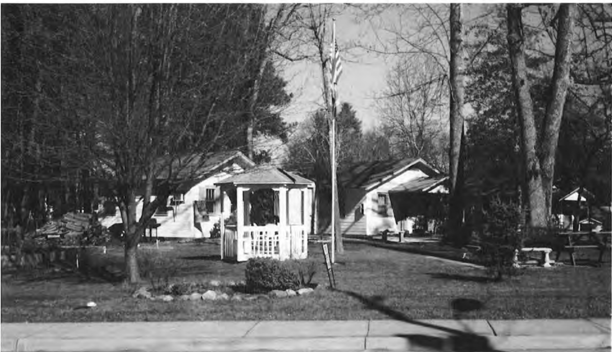
Villa Capri Cottages (former Carolina Court), 920 Greenville Hwy, main residence, view to east
