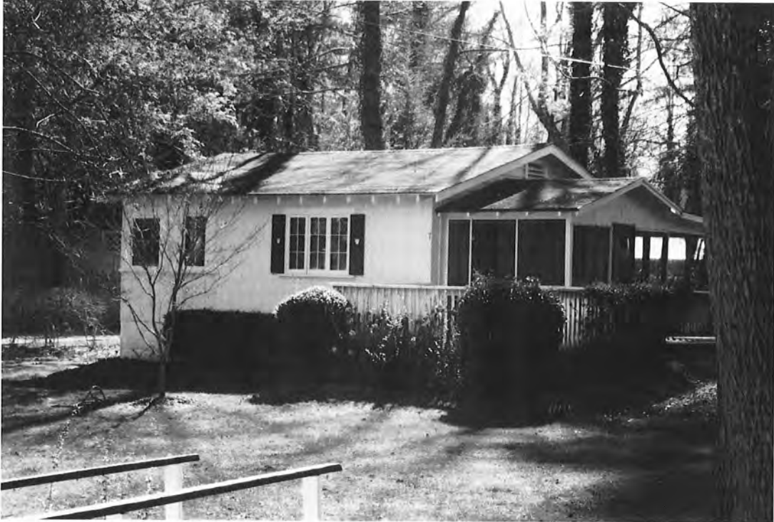
Cottage #7, 28 Drifting Cloud Lane, oblique front view to southeast
