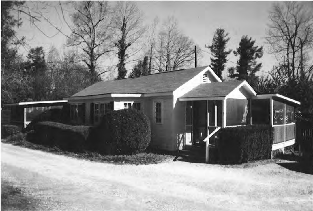
Duplex Cottage #1-2, 124 Ivy Brook Lane, oblique front view to northeast
