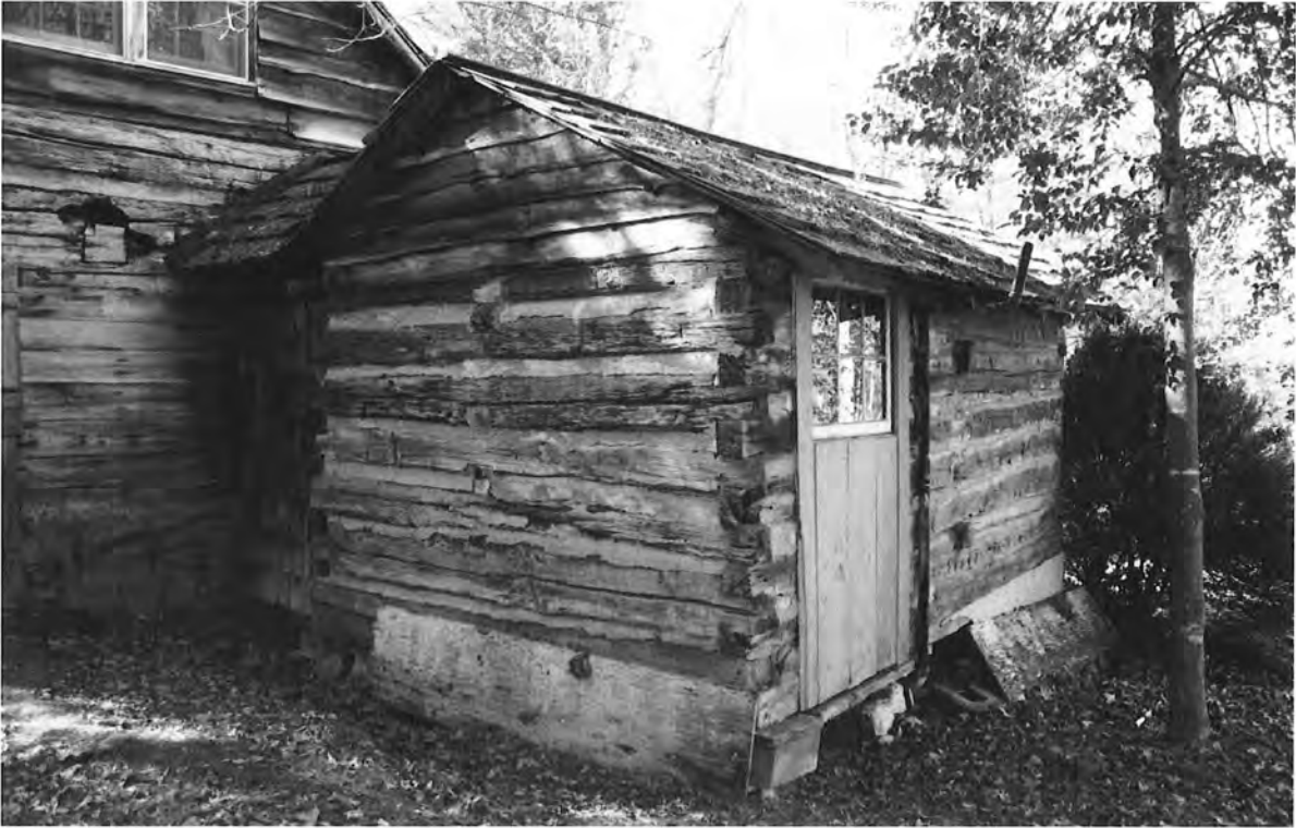
Loom house wing, oblique rear view to northwest
